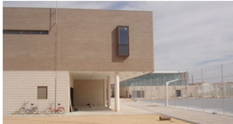
Secondary school in the town of Villa de Don Fadrique, Toledo
